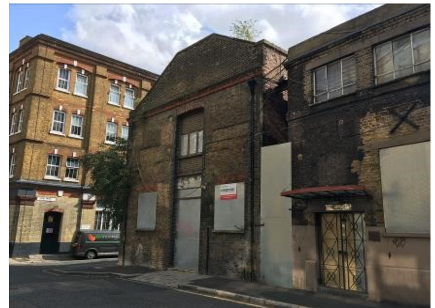
Figure 17: Poorly maintained warehouse on Sanctuary Street
