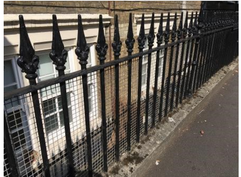
Figure 18: Railings on Mint Street
